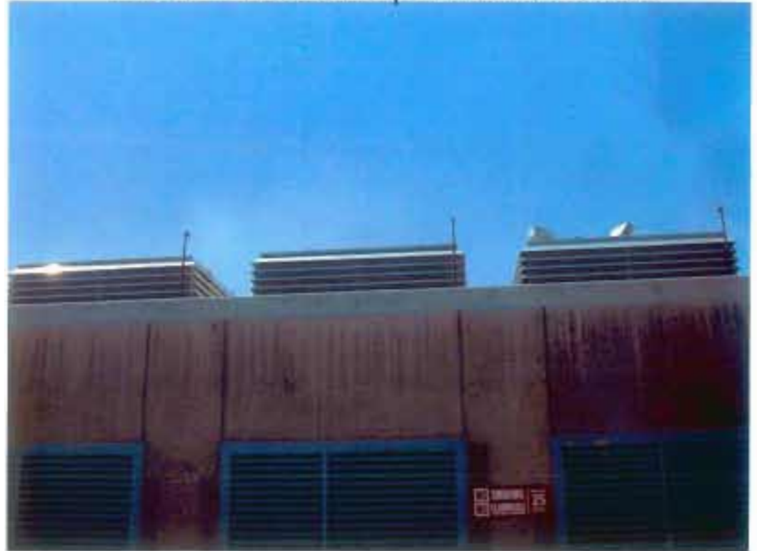
2721-Z inlet and penthouse vents
