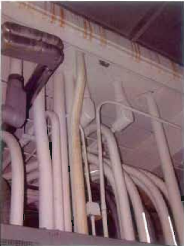
Conduits at 291-Z switchgear showing evidence of past water exposure
