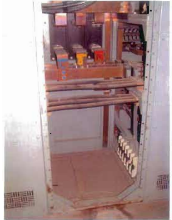
291-Z Switchgear enclosure. Lower panel below water stains
